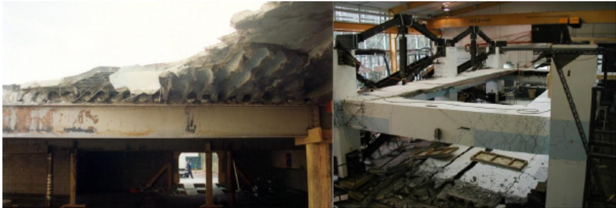
**Figure 2: Photographs of damage to precast concrete floor systems. Left shows the Meadows Apartment Building, California, as a result of the 1994 Northridge earthquake. Right shows Matthews super-assembly specimen at the completion of the Phase 1 testing. Note the specimen’s floor dropped out at a low seismic load with little damage to the surrounding frames.**
